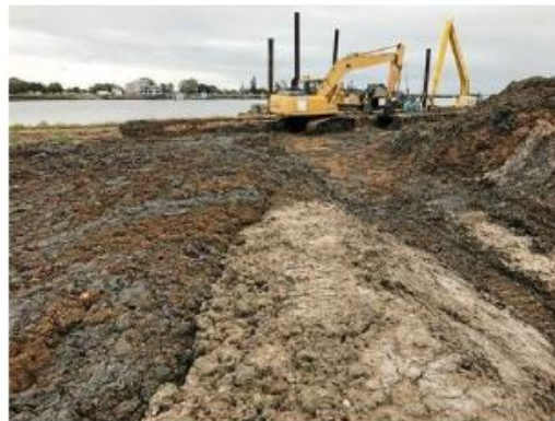
📷 Dredging work is well under way at the marina.
