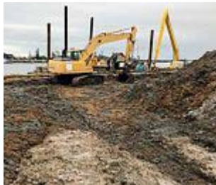
Dredging work is well under way at the marina.
