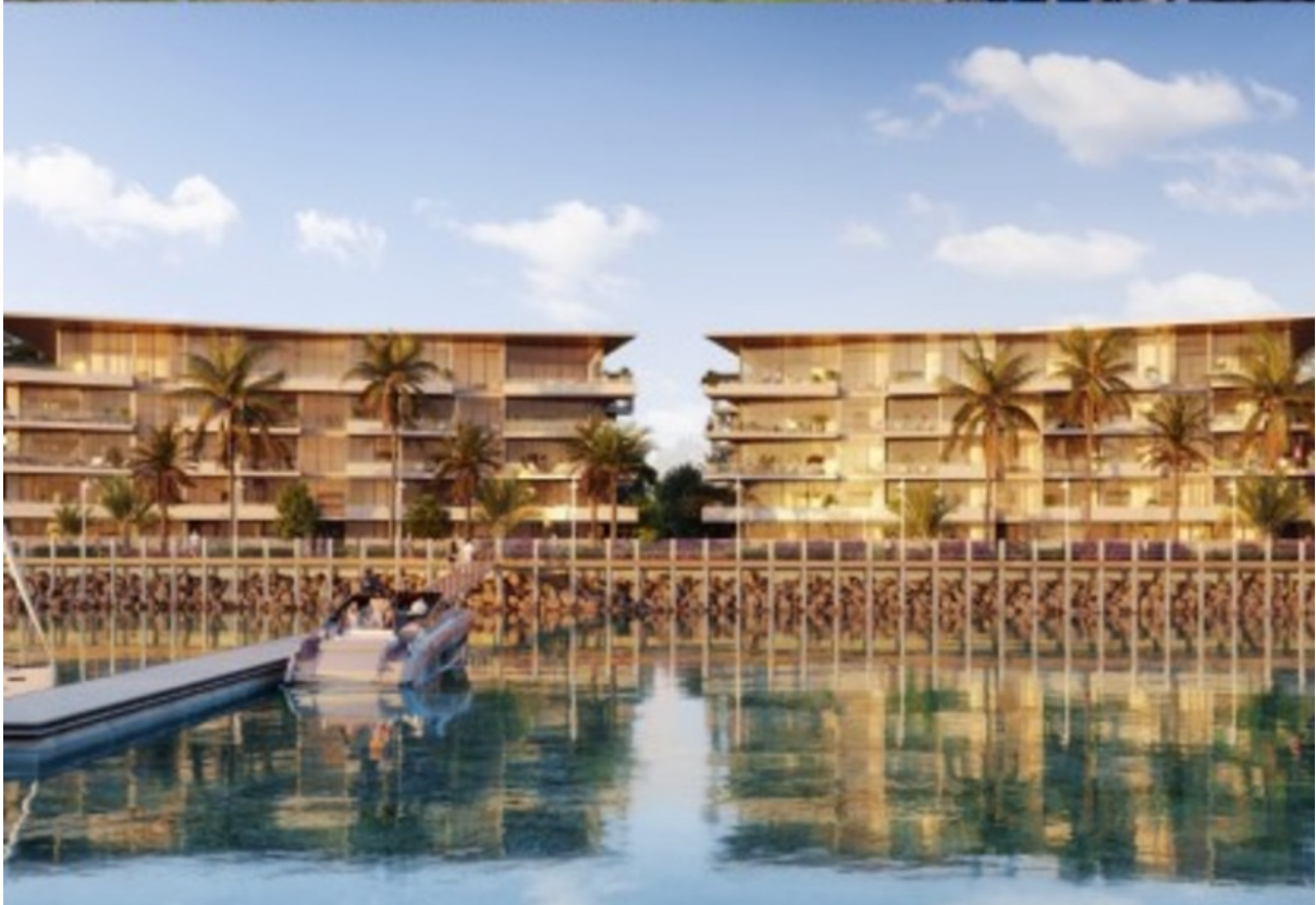
Work has begun on the new Gateway Marina, with an artist's impression showing the future development design.
